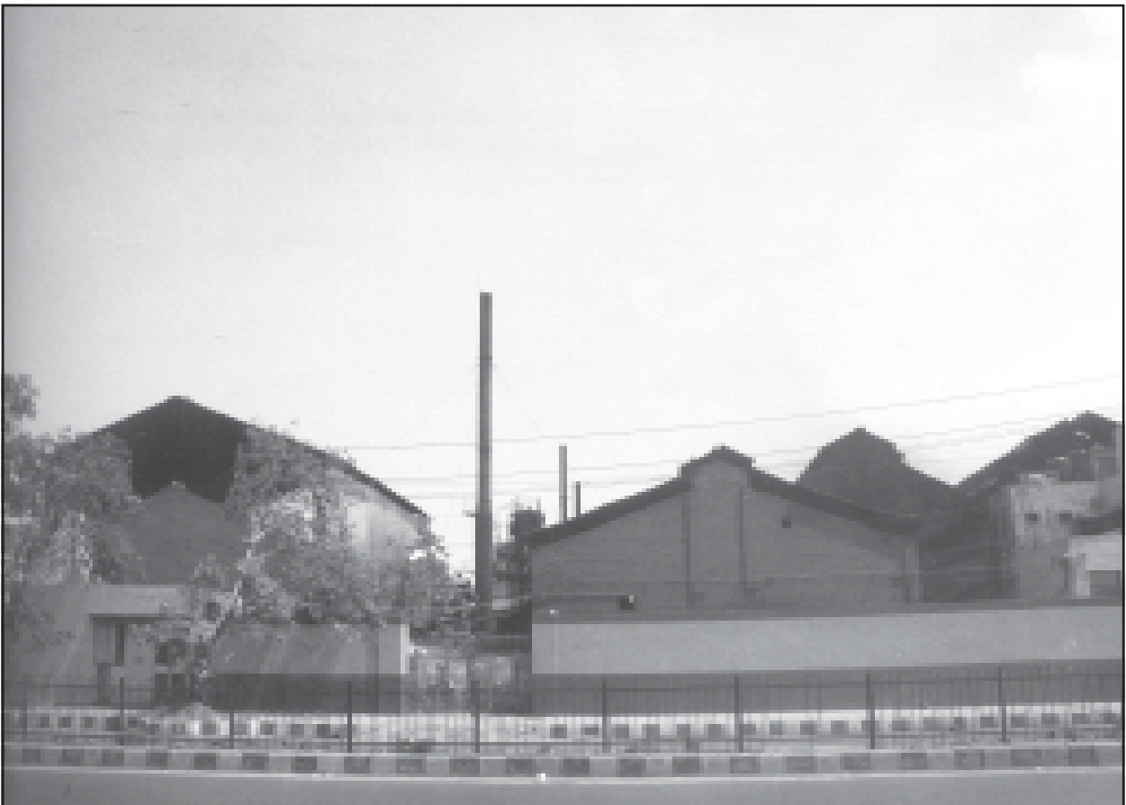
Industrial area, Mayapuri
